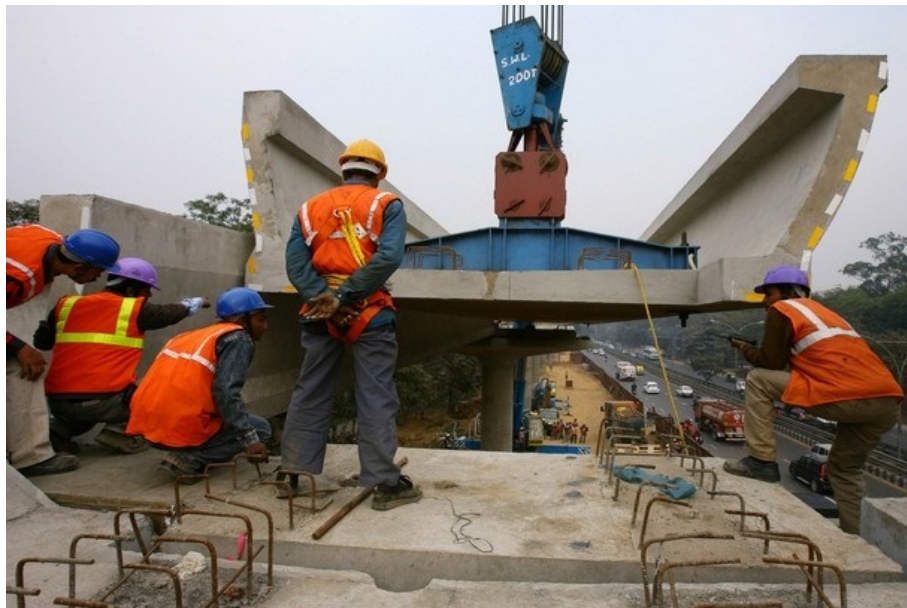
Figure 1.9: Erection of U-shaped girder
